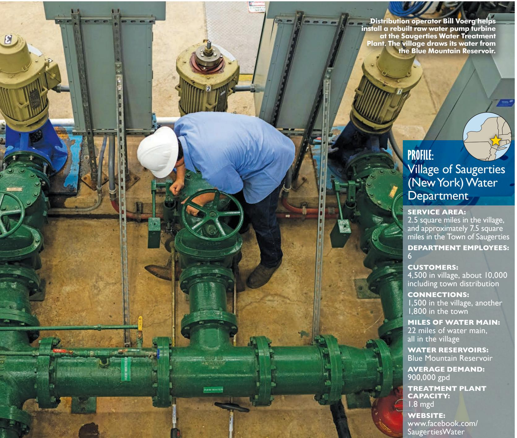
Distribution operator Bill Voerg helps install a rebuilt raw water pump turbine at the Saugerties Water Treatment Plant. The village draws its water from the Blue Mountain Reservoir.
